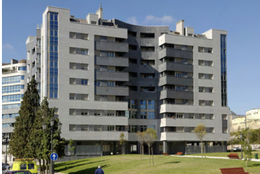
Facades constructed with different stone varieties
